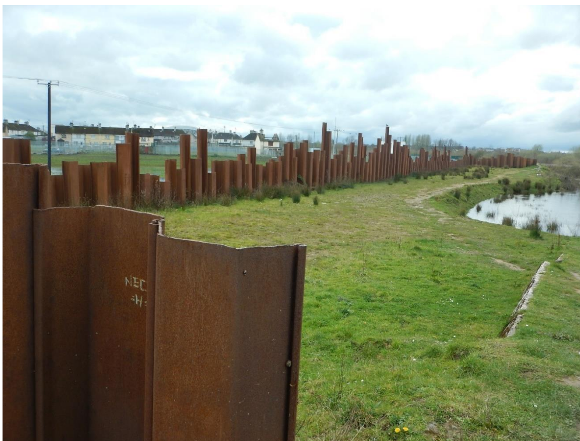
Figure 3-11: Sheet piling and bare ground pathway
